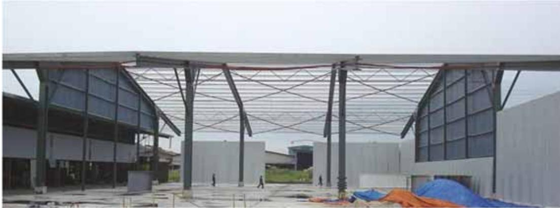
**Fig. 8.** UHPC portal frame (before completion at year 2008).
