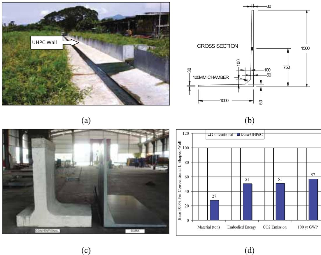
**Fig. 12.** (a) 90 m long monsoon drain using UHPC retaining wall; (b) cross-section detail; (c) comparison of conventional precast L-shape retaining wall with UHPC wall; and (d) environmental impact calculations of UHPC retaining wall.
