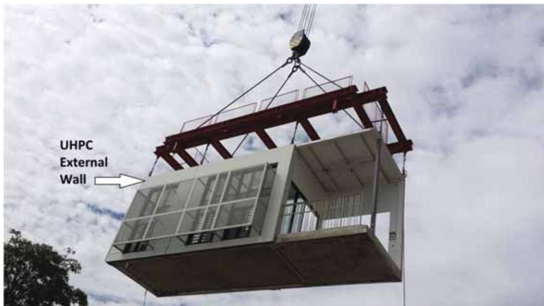
**Fig. 14.** Lifting of PPVC unit.
