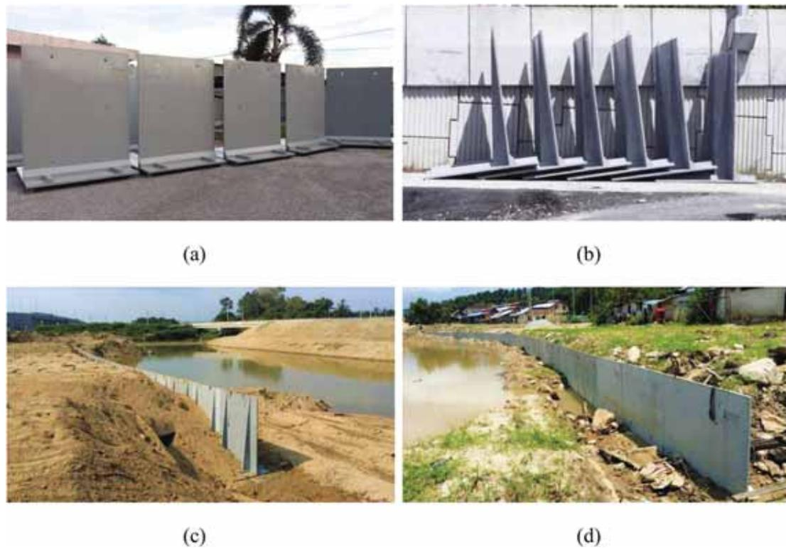
**Fig. 10.** (a) and (b) UHPC retaining wall at storage yard; (c) and (d) 120 m long retaining wall installed for slope and river protection.
