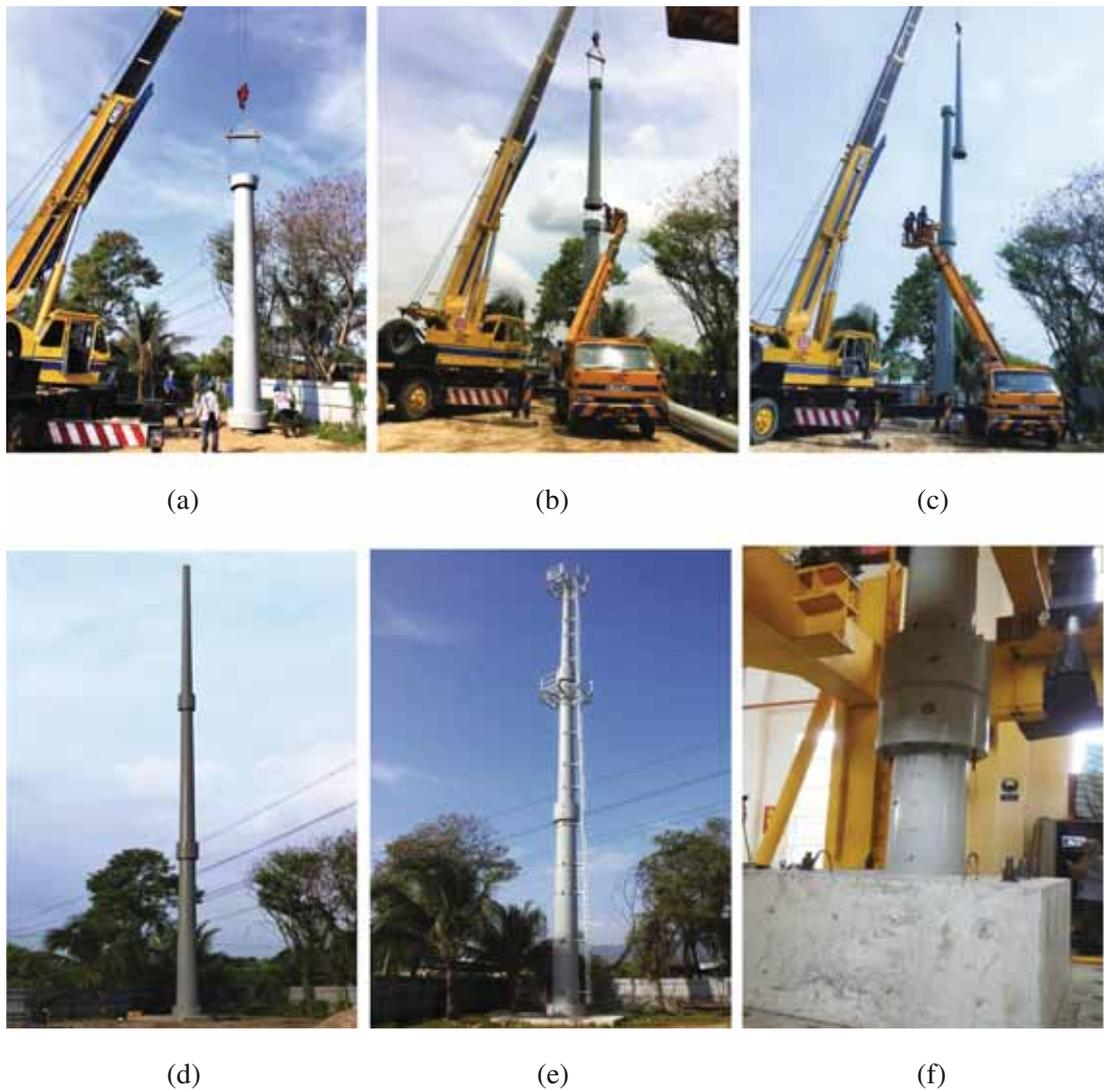
**Fig. 7.** Lifting/assembly of (a) first bottom-segment; (b) second middle-segment; (c) third top-segment. (d) Fully assembled UHPC prestressed/precast tower with (e) ladder and working platform installed. (f) Full-scale cyclic loading test on the segmental epoxied joint at the structural laboratory of Universiti Putra Malaysia.
