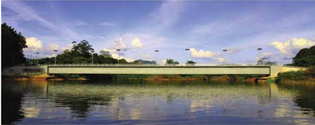
**Fig. 6.** 100 m long single span Batu 6 Bridge.
