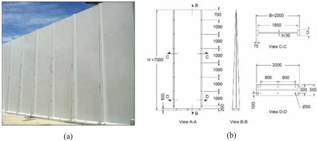
**Fig. 11.** (a) UHPC anti-climb wall and (b) detail of wall panel.
