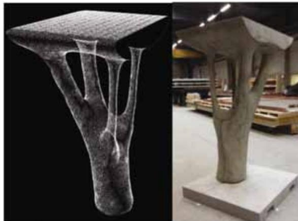
**Fig. 17.** (a, b) Optimized column designed and manufactured by CNC milling
