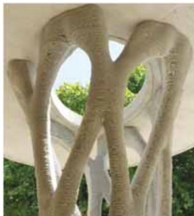
**Fig. 18.** A similar biomimetic type of column printed by XtreeE (Gosselin et al. 2016)
