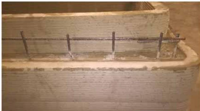
**Fig. 13.** Hybrid solution: printed concrete as lost form work for conventional cast concrete with reinforcement.
